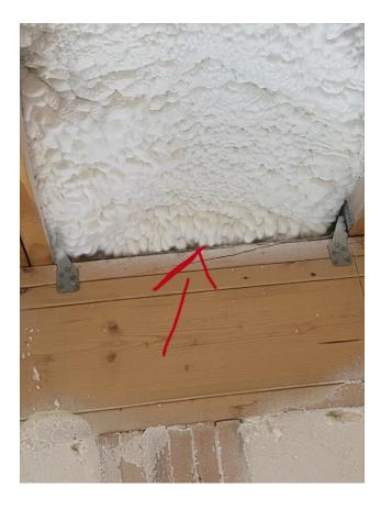
Fortunately, this is an easy problem to solve. Simply make sure that lower flange of the cardboard is installed as far back as possible, or our preferred approach, just attach the baffle to the outside of the wall.
