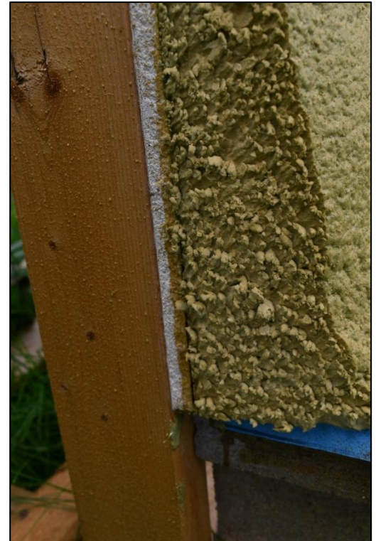
Figure 7. SealTite One with colour faded by UV exposure after approximately 3 weeks.
