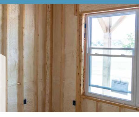
Carlisle spray foam insulation applies smooth, expands into hard-to-reach crevices, and provides optimal R-value and air sealing to support today's challenging building code environment.
